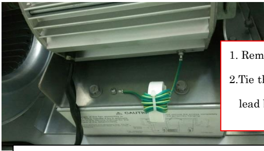
Photo of motor earth lead before repairing
